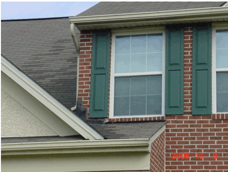
Photo 2 - The front downspout upper level should be extended around the corner. The present arrangement offers a greater potential to leak at the flashing. Also, a deflector attached to the gutter at the valley will prevent overflow during heavy rains.
