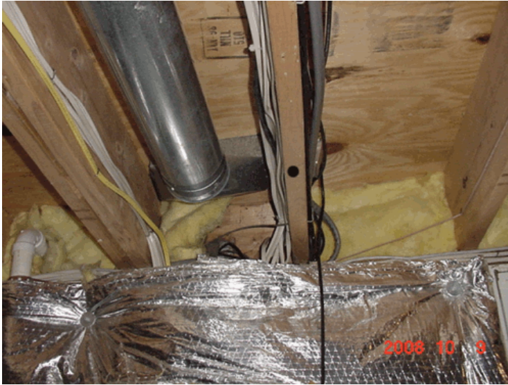
Photo 4 - All exterior penetrations should be sealed. Also, the sill plate and box plate (rim joist), should be sealed using spray foam insulation.
