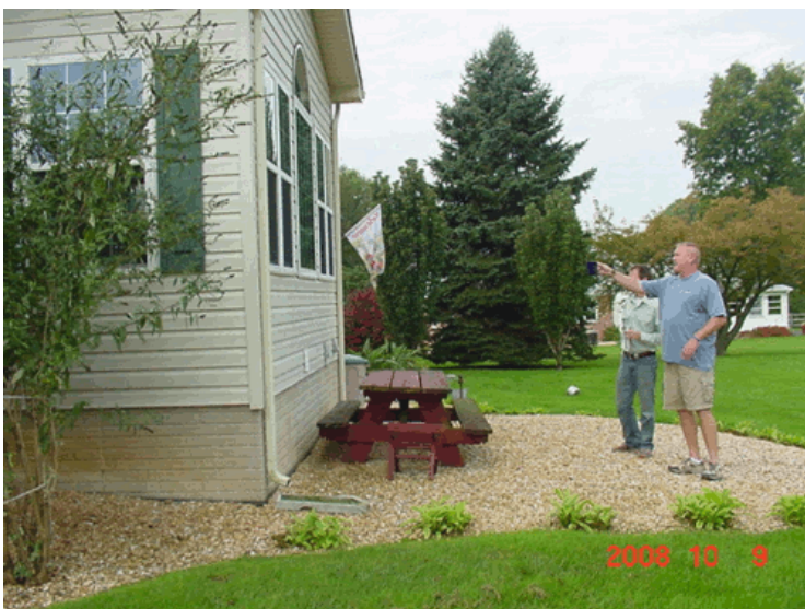
Photo 2 - The front downspout upper level should be extended around the corner. The present arrangement offers a greater potential to leak at the flashing. Also, a deflector attached to the gutter at the valley will prevent overflow during heavy rains.
