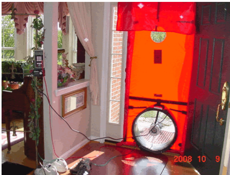
Photo 9 - Arrangement of the blower door test includes an adjustable fan with a differential pressure gauge adjusted to a specified level.
